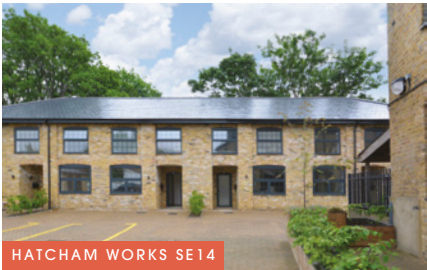
Hatcham Works SE14 Beautifully restored Victorian warehouses in the Hatcham Park Conservation Area, comprising 6 houses and 10 apartments.
